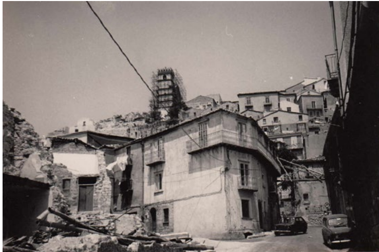
Earthquake in Irpinia, municipality of Castelgrande, Potenza (November 1980).
