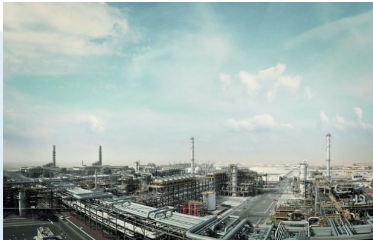
Habshan 5 - Gas Field Development Project - Sulphur Recovery Units & Acid Gas Removal Units, 2009-2013
