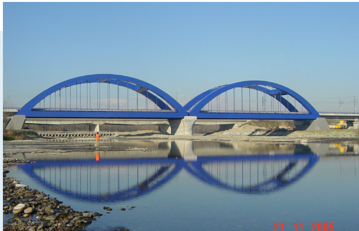
Double viaduct over the Dora Baltea, November 21 st 2005
