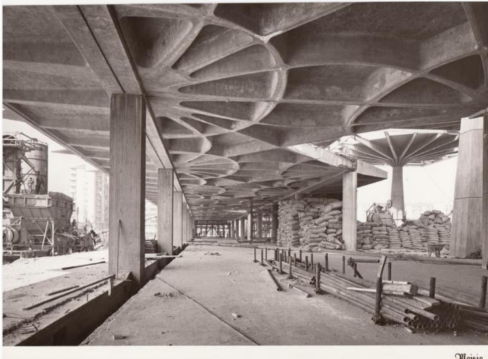
The Palazzo del Lavoro, in which the engineer Gino Covre and architect Giò Ponti are also involved, is a true masterpiece of modernity and beauty. It looks like a squared-off spaceship with its sixteen 25-meter-high "large umbrellas," each consisting of a steel pillar from which steel arms protrude to support the building's roof.
